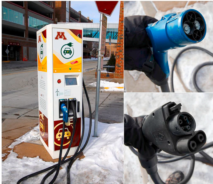
Fig. 21. An example of a Level 3 DC Fast Charging station with CHAdeMO (top right) and CCS (bottom right) adapters. "umn-chademo-and-ccs-charger" by Mulad is licensed under CC BY 2.0.
